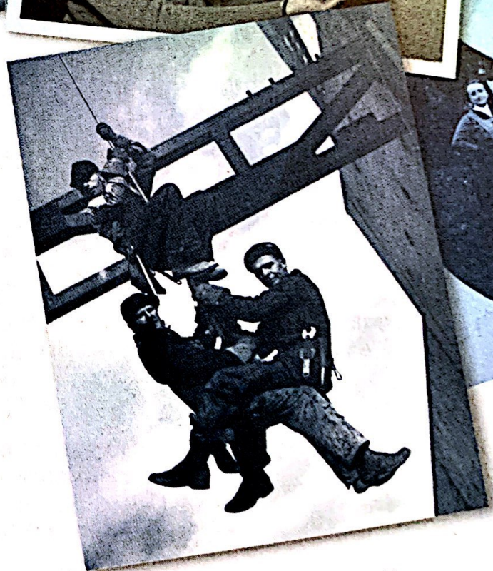
Relief workers on a cable during the construction of the Fort Peck Dam, 1936
