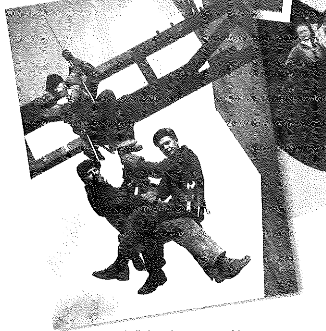
Relief workers on a cable during the construction of the Fort Peck Dam, 1936
